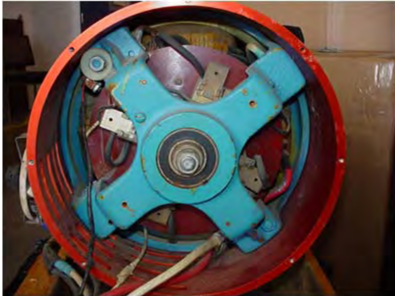
Back End View of the "Start Motor"
